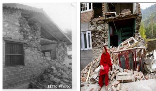
Figure 1. Failure in masonry brick houses
